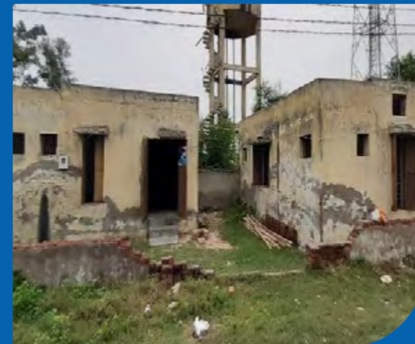
Before and after pictures of the renovated Aanganwadi at Jalalpur
